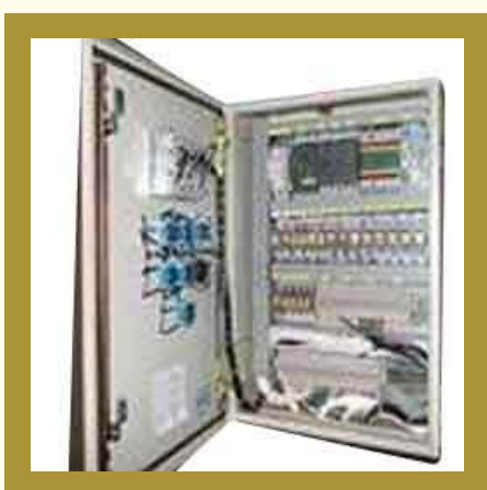
Panel Manufacturing & Repairing(Rectification)
